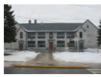
ANNVILLE ELEMENTARY SCHOOL (1)
