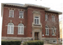
LEBANON VALLEY COLLEGE CARNEGIE BUILDING (22)
