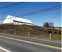
IRON FURNACE / CHARCOAL BARN / SPRING HOUSE (37)
