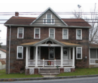
OFFICES FOR FURNACE OPERATIONS (35)
