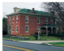
DR. STAUFFER HOME AND OFFICE (14)
