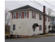
CONEWAGO VALLEY GRANGE HALL (19)
