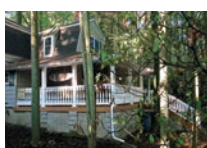
PENNSYLVANIA AVE. COTTAGES (17)
