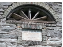
HANSHAW LIMESTONE BANK BARN (29)
